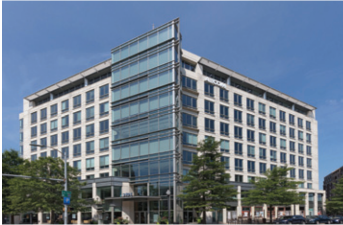
The Hartford Building at Clarendon Station
